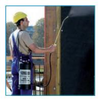
Even adequate to the heaviest duties: In building trade the models 405 T Profiline and 410 T Profiline are applied in particular for the dispersion of mould oil.
